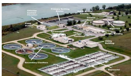
Figure 6.4.1 A Typical Biological Sewage Treatment Plant
